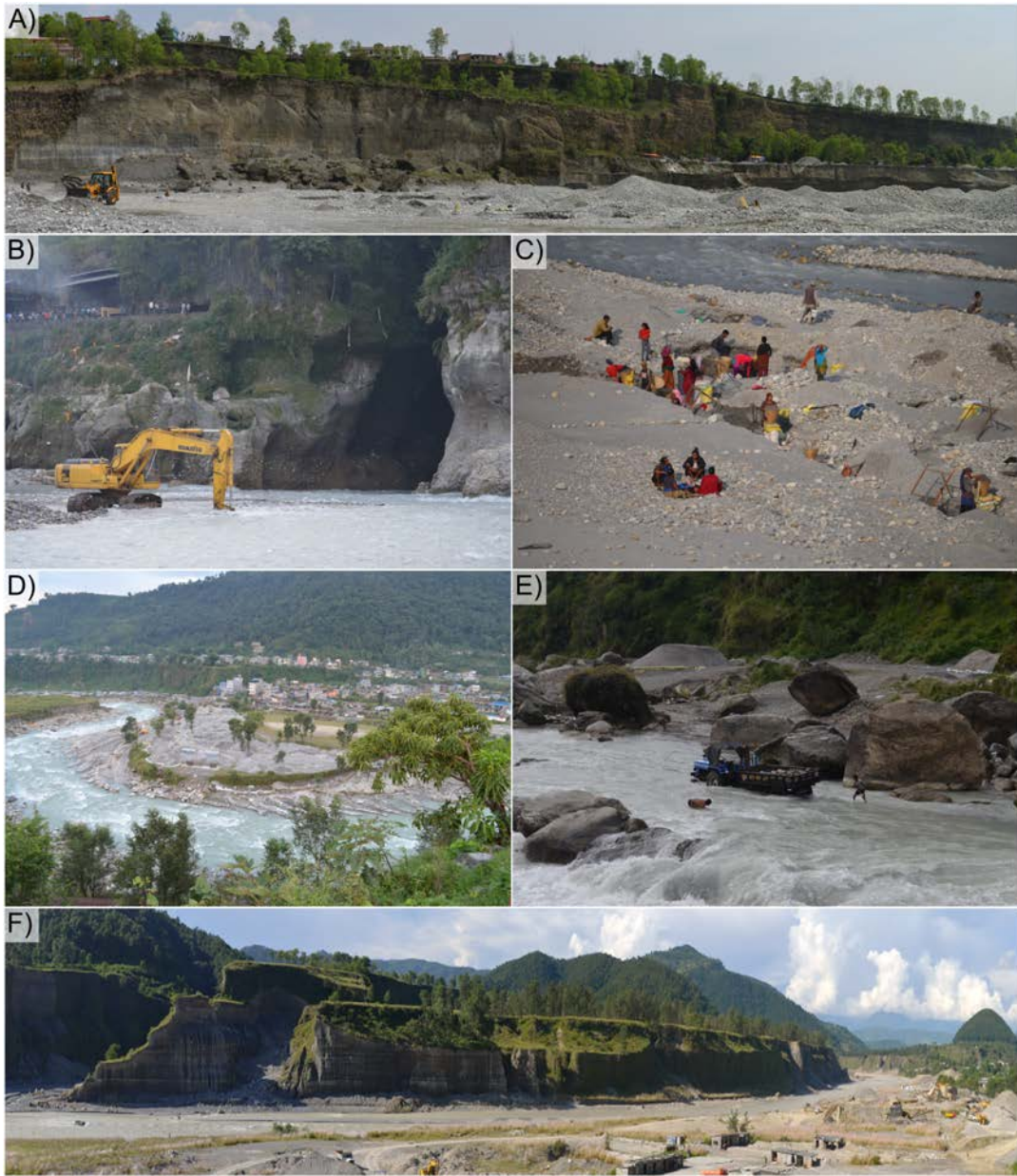
Figure 1.4.: Field images of excavation work along the main river. A) Panoramic view in the Ramghat area (see Fig. 3.1 for the location) in the center of Pokhara city. Seti Khola runs along the outcrop in the back while hundred of people screen, sort, and carry gravels ( C ) from sand to boulder sizes. B) Same location as A) and C), at the outlet where the Seti disappears in a bedrock gorge. D) Place for river mining north of Pokhara city. Groins are set to trap sand particles carried by the river during the monsoon season. E) Groups of locals collect river clasts in the Seti Khola. Note the boulders outsizeing the tractor. F) Downstream at the confluence to Pudi Khola (Fig. 3.1), one of the biggest construction areas, where machines sort gravels from the channel beds.
