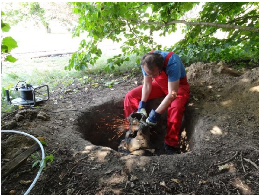
Fig. 1.12: Cut-off of the well head by Dr. B. Norden (9/02/2011).
