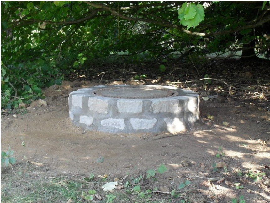
Fig. 1.16. Manhole cover put in place by the Geological Survey and the Administration des Ponts et chaussées (Luxembourg) and now securing the Mersch borehole.
