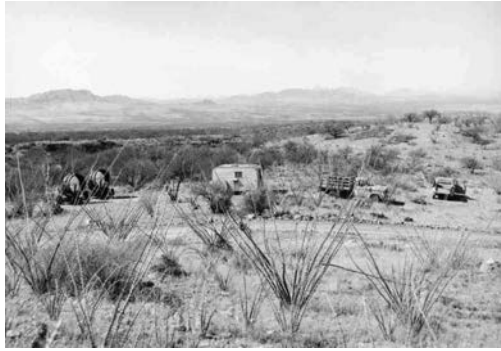
(a) The first TeV gamma-ray observatory in the United States consisted of two searchlight reflectors from World War II with a size of 1.5 m each. They were operated in the year 1967. Image from Weekes (2008).
