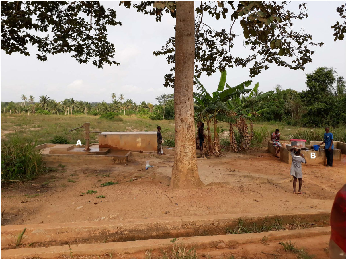
Figure 1.1: Sources of water supply in the Pra Basin include mechanized boreholes fitted with hand pumps for community water supply with depths usually less than 60 m (A) and hand-dug wells usually completed to a depth of less than 20 m (B). Picture taken on March 17, 2020.
