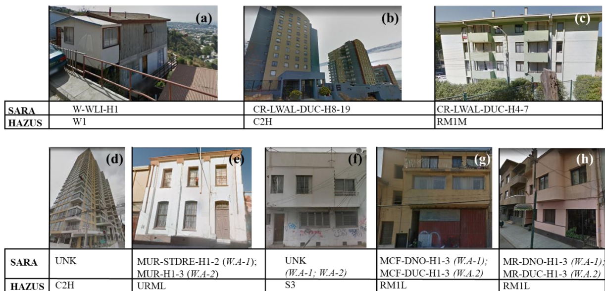
Figure 2-3. Pictures of some selected buildings' façades surveyed in Valparaíso. Their classifications in terms of the SARA and HAZUS schemes are displayed considering the two weighting arrangements presented in Table 2-3. ©Google Street View, 2021.
