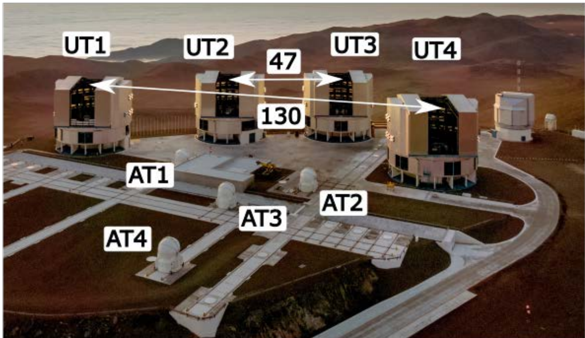
Figure 1.3: A photograph showing the very large telescope interferometer (VLTI) facility situated on Cerro Paranal in the Atacama desert of Chile. The four unit telescopes (UTs), each having a diameter of 8 m, are marked in the photograph. The longest and shortest baselines formed by the four UTs are shown in meters. The four auxiliary telescopes (ATs), each having a diameter of 1.8 m, are also marked. The UTs are fixed, but the ATs can move along the white tracks to increase the u-v coverage and, at the same time, maintain non-redundancy in combining stellar light. Image retrieved from Ref [6].
