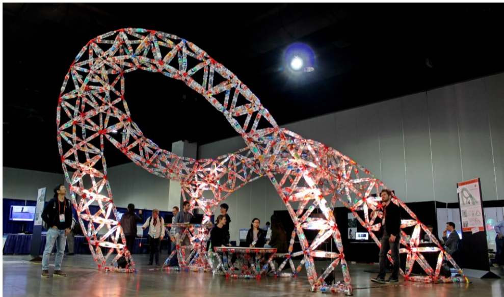
Figure 4: TrussFab pavilion created from ~1200 PET bottles and 119 3D printed hubs, presented at CHI'17, Denver, USA.
