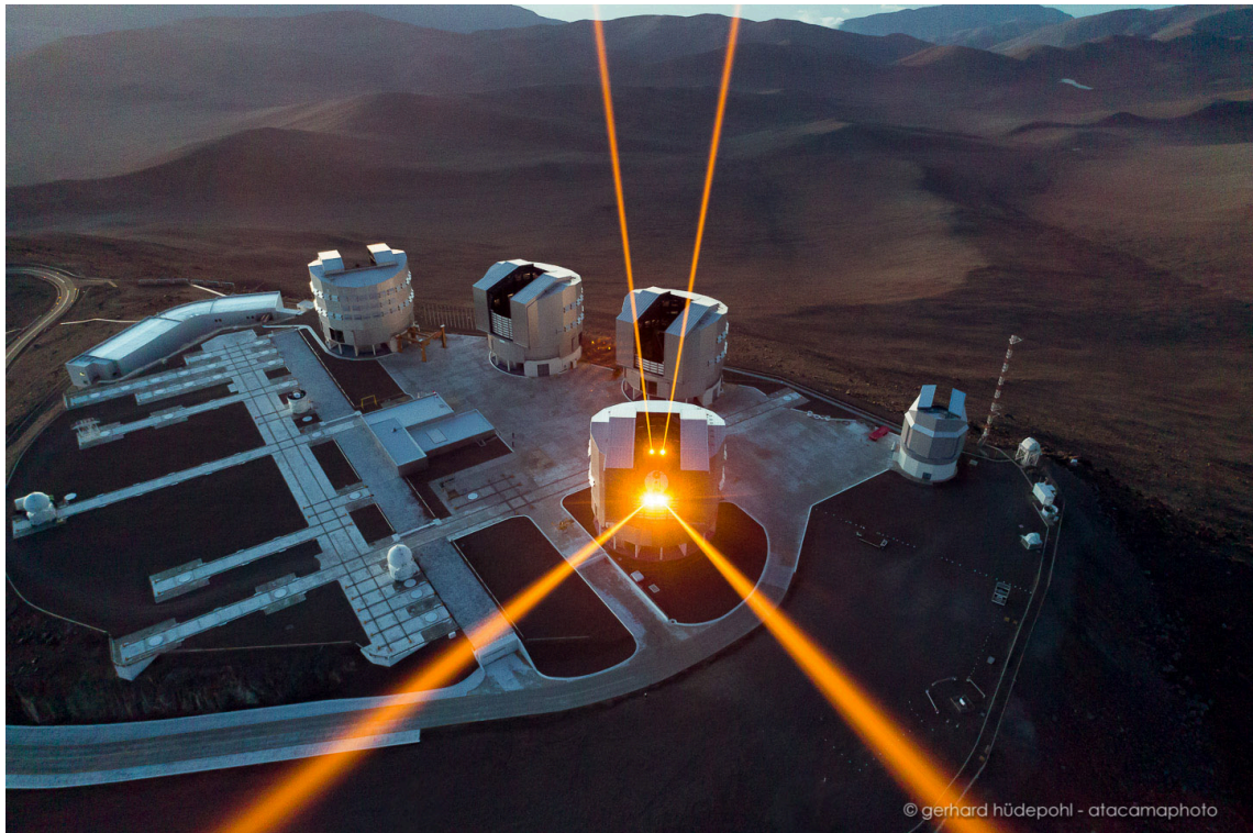
Yepun, where MUSE is installed, with its four Laser guide stars. Credit and licence: European Southern Observatory / Gerhard Hüdepohl ( atacamaphoto.com ).
