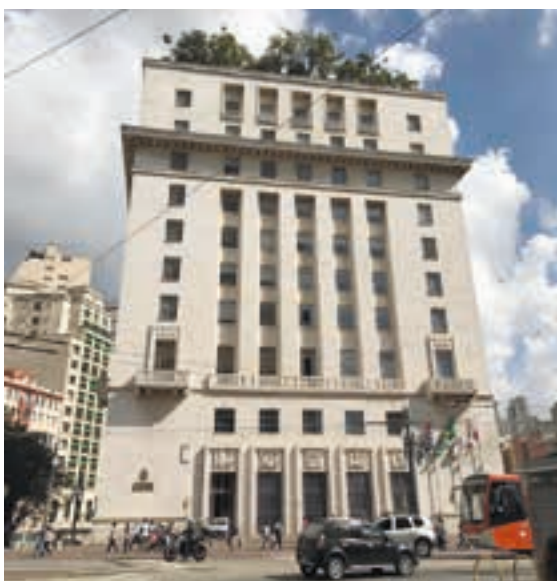
The municipal administration of São Paulo sets a good example of “Urban Greening” with its rooftop garden.
