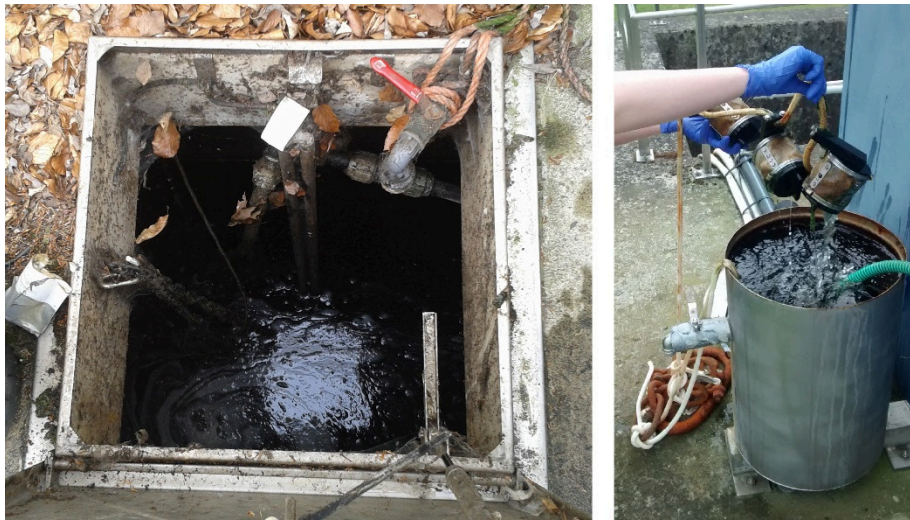
Figure 3. Pictures showing the exposure locations of the second experiment of study I inside a WWTP. Station 6 (left) is situated after the last sedimentation tank and station 7 (right) after the final treatment with an oxygenated biofilm reactor.
