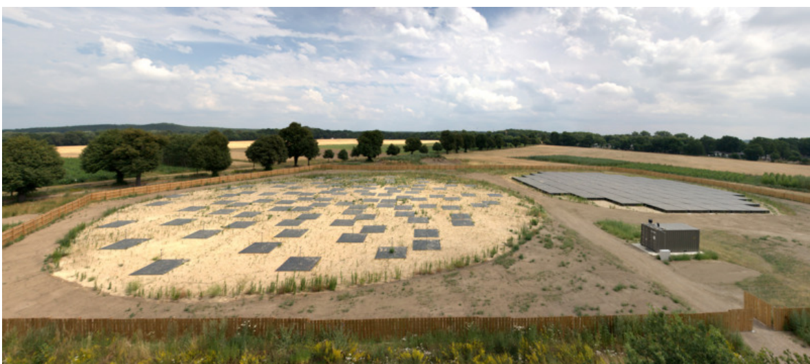
Figure 4.3: International LOFAR station (DE604) in Potsdam-Bornim with the low- and high-band antenna fields to the left and right respectively. The container in the front right houses the receiver and computer electronics and the connection to the Internet.
