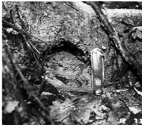
Figure 3. The outlet of pipe 2 (see Figure 2 for location).
