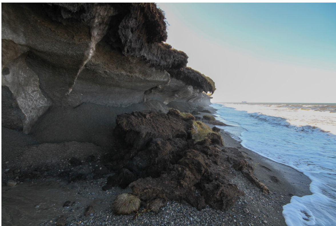
Figure 3.7: Thermo-erosional niches building an overhang at Stokes Point where the coast retreated by up to 20 m between 2012 and 2013.
