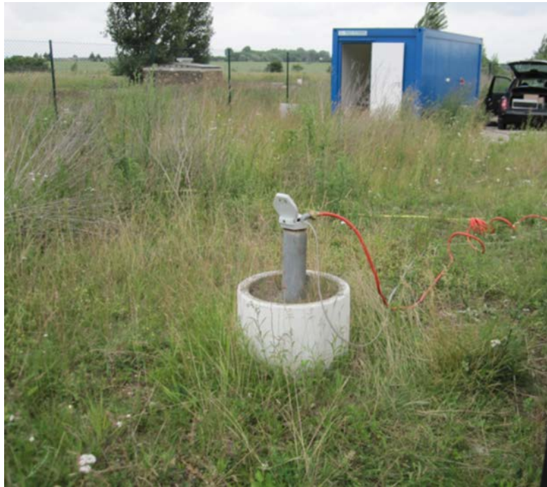
Figure C.7.: Image of the extraction well during the experiment.
