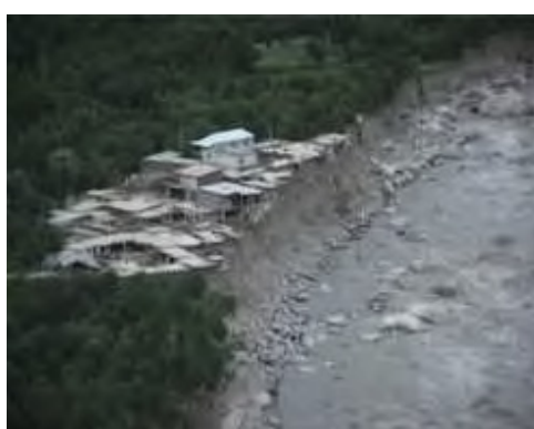
Figure 20: 2005 Flood: Damage to Leo Village
