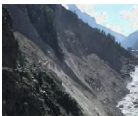
Figure 21: Loss of road and landslides
