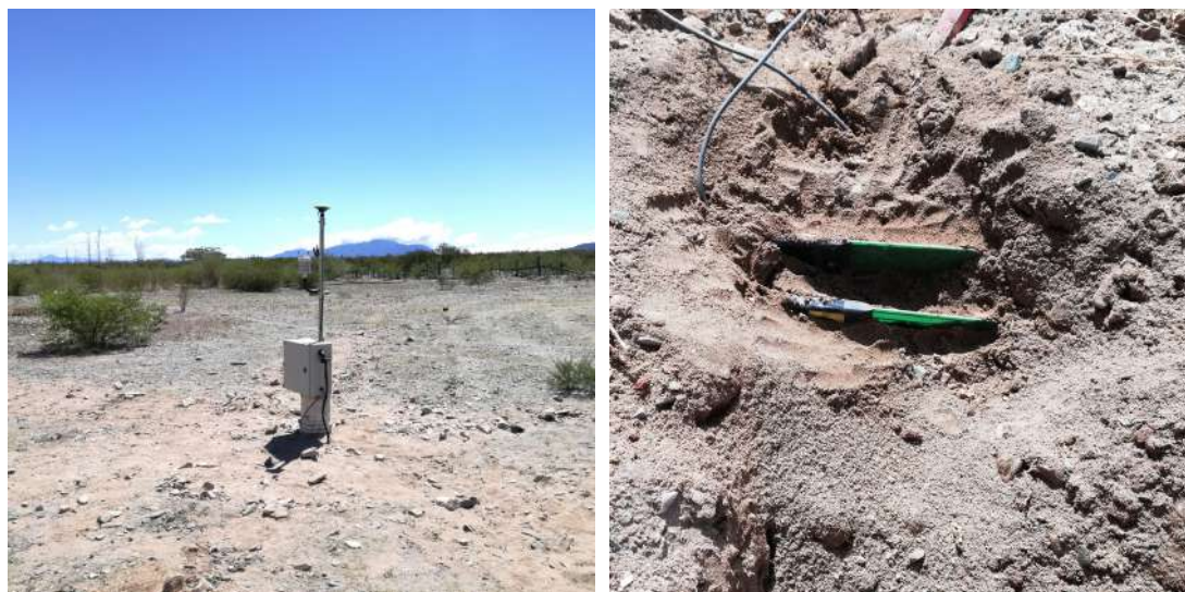
Figure 7.4: Tolombon station. Left: GNSS and meteorological equipment installed on a 2 m pole. The metal box includes all necessary instrumentation (Looking angle in the north direction). Right: Soil vertical profile and two TDR-FDR probes arranged at distinct depths. In the photo is shown the top-layer soil composition, including the organic matter, the different size granules, and pebbles.
