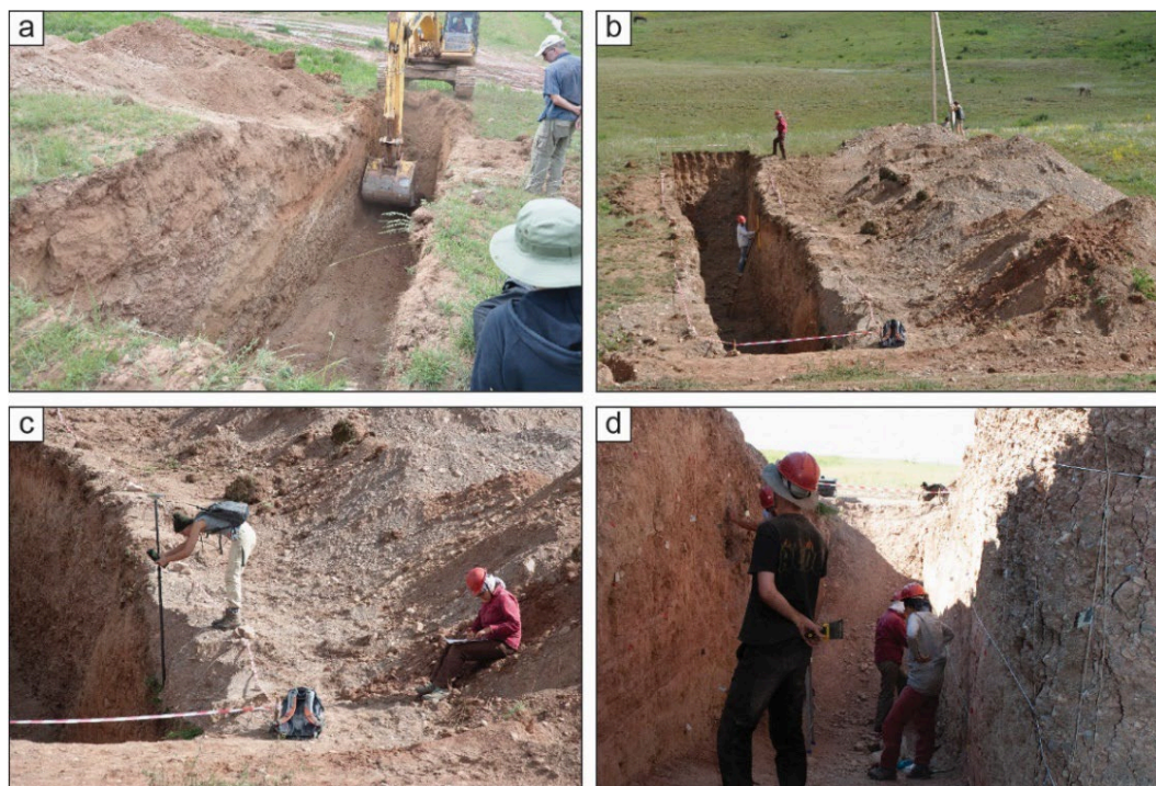
Figure 3.5 The Achyk-Suu trenching site, a) excavation; b) single-slot trench across a 7-m-high thrust-fault scarp; c) reference-grid measurement with dGNSS; d) view of trench interior.
