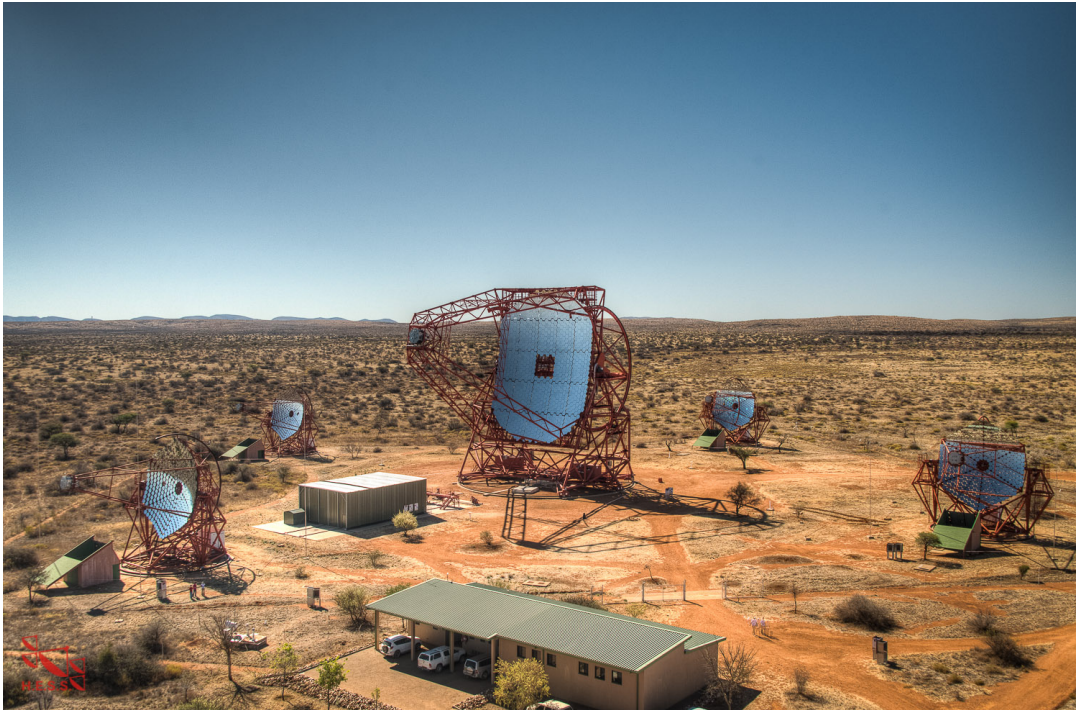
Figure 2.5: The High Energy Stereoscopic System (H.E.S.S.) in the Khomas Highland of Namibia [130]. CT 1 - 4 are located in the corners of the array and CT 5 is in the middle. In front of each telescope, there is a camera shelter, in which cameras are secured during the day or bad weather. A control building, from where the telescopes are operated, is seen in the bottom of the photo. Credit: H.E.S.S. Collaboration, Christian Föhr.
