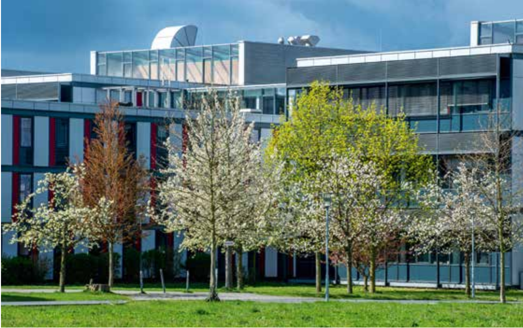
Building 25 (left) and Building 26
