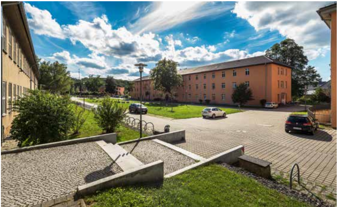
View of the former roll call square from Building 5
