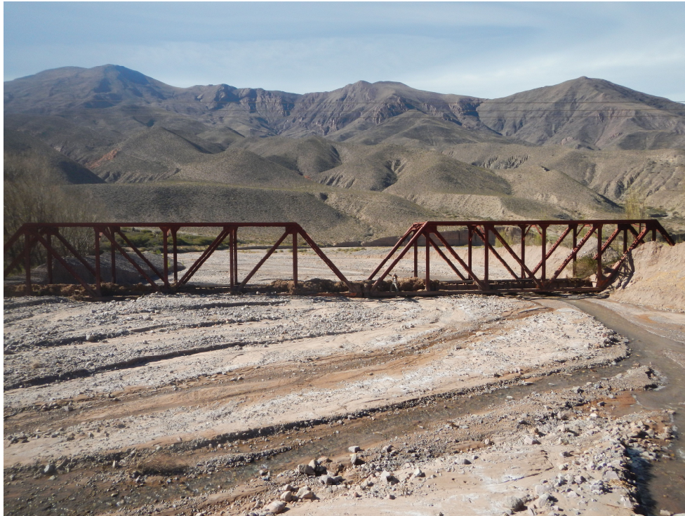
Fig. 1.2 Photo of the train bridge crossing the Yacoraite river in the Quebrada de Humahuaca. Due to bed elevation rise and repeated destruction of the tracks, the train tracks were abandoned in the 1990s.
