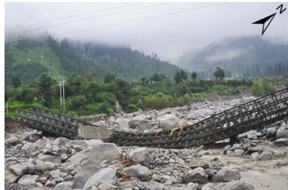
Figure 1.10: View of the Beas Valley. Beas River at Palchan with bouldery deposits after intense rainfall in the Rothang area in the night of August 3th to 4th, 2012. The resulting flood obliterated houses and roads at the riverside and a bridge between the Rothang and Manali.
