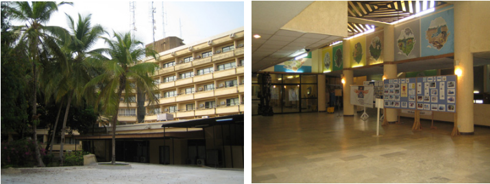
Figure 14: UNIOSIL building, Freetown Source: Author (2008)
