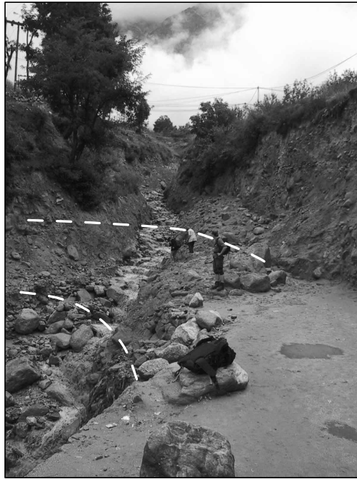
Figure 3.10: Remnants of a debris-flow in the village of Sangla, Baspa Valley during the 2002 AMY (31.8.2002). White dashed lines indicate location of destroyed road. Note levee material related to debris flow showing the thickness of the flow.
