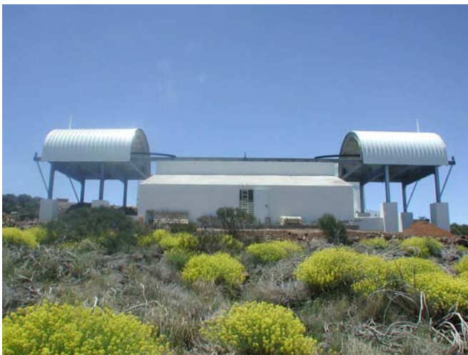
Figure 3.2.: Outside view of the STELLA building in construction. The roofs are fully open, visible are the blocks at the end of the rails and the black energy chains used for power and signal cables to the moving roof.
