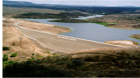
Figure 4.3 View of the Benguê reservoir in 2002.
