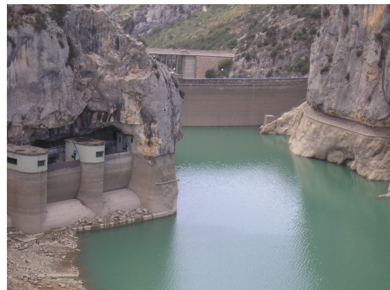
Figure 4.18 View of the Barasona dam and its radial crest gates.
